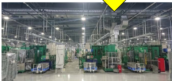
Factory floor after equipment installation
