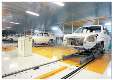
Conveyance system for automobile manufacturing line
