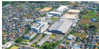
Photograph is of current Saitama Plant
